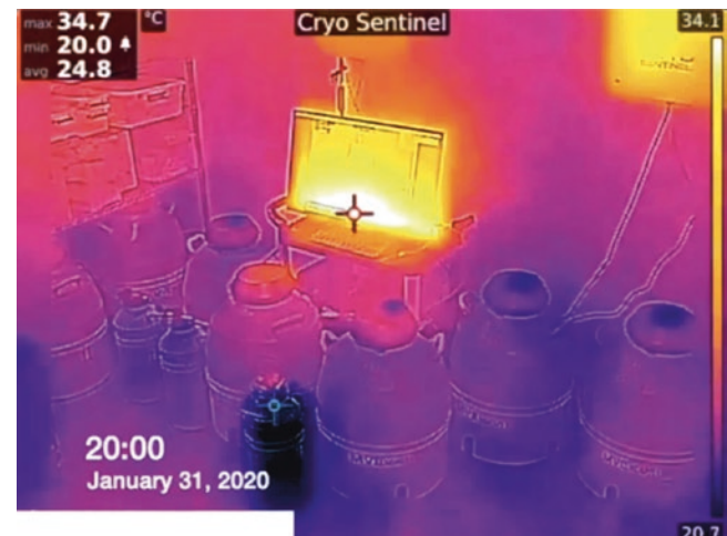
Fig. 46.3 A failing dry shipper showing signs of vacuum failure with CryoSentinel thermographic monitoring
